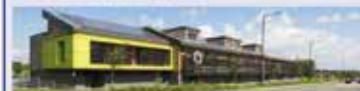
Filwood Green Business Park, Bristol - An example of an environmentally friendly employment development
