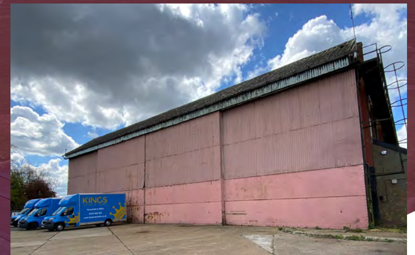
Hangar 1 - Bat Roost Potential
