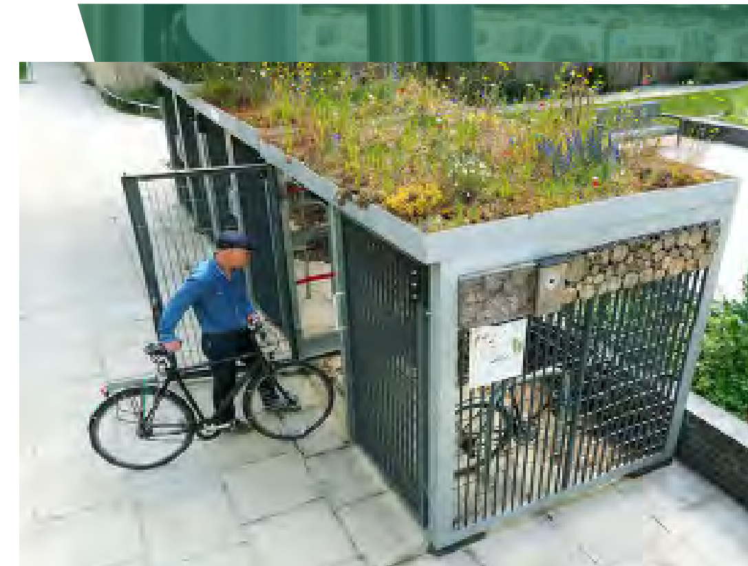
Cycle store with green roof
