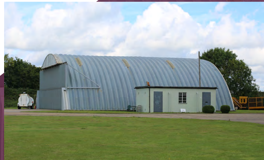
Existing hanger building located airside
