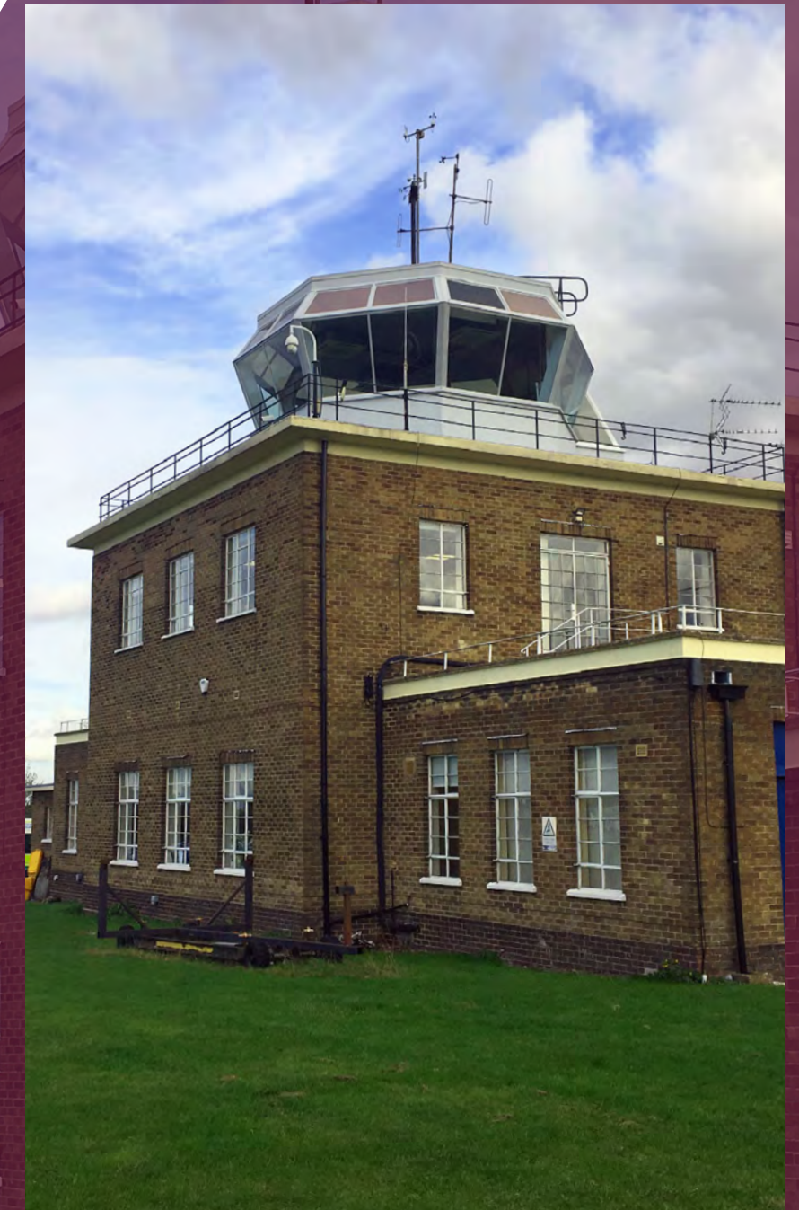
North Weald Airfield Control Tower
