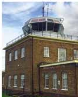
North Weald Airfield Control Tower
