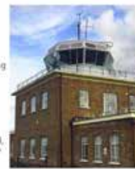
North Weald Airfield Control Tower
